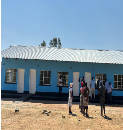
Jondale Primary School block (Mhondoro Ngezi)
