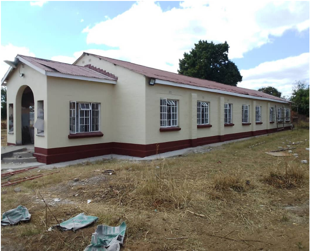
Beatrice National Rehabilitation Centre
